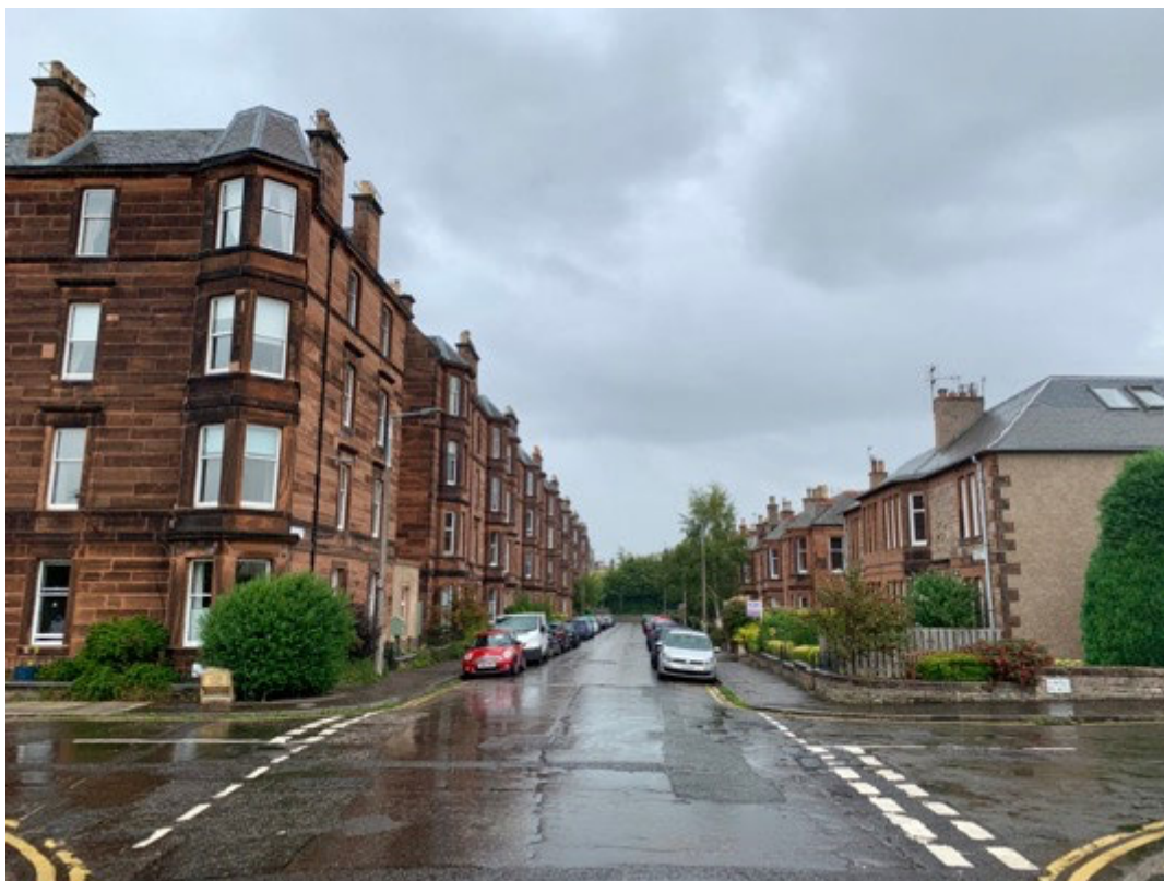
Photo 1 – View North East along Macdowall Road with applicant's house on right.
