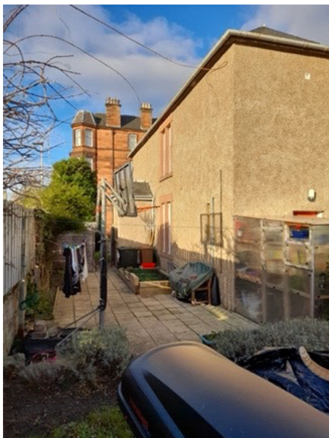
Photo 4 – View towards side of applicant’s house from the rear, showing the side windows in full sun.
